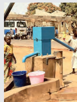
Rehabilitation and replacement of a broken hanpump by the BluePump.
