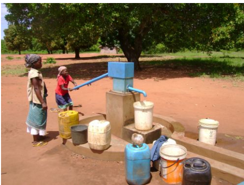
Bluepump at 65m deep on rehabilitated borehole, Unicef project Mozambique
